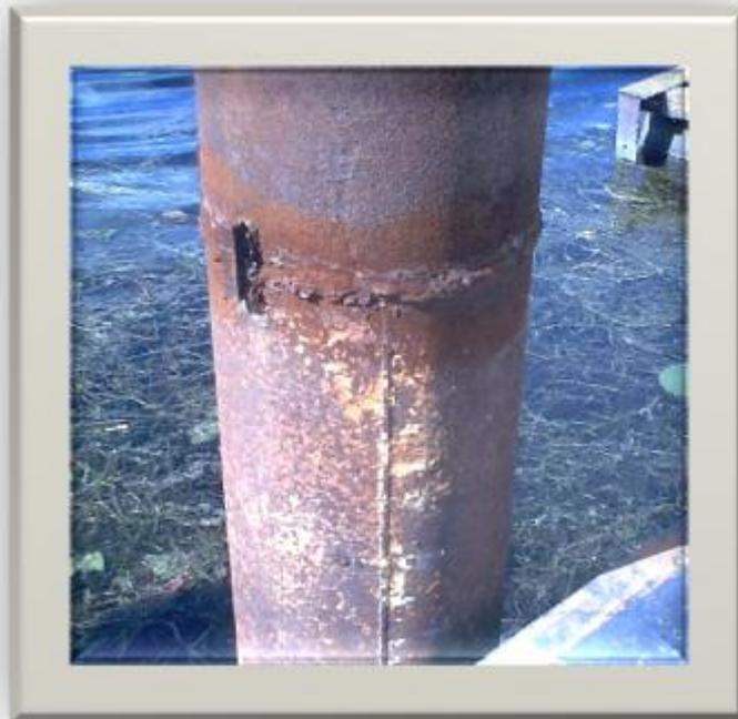
**Figure II.8-** La corrosion uniforme
